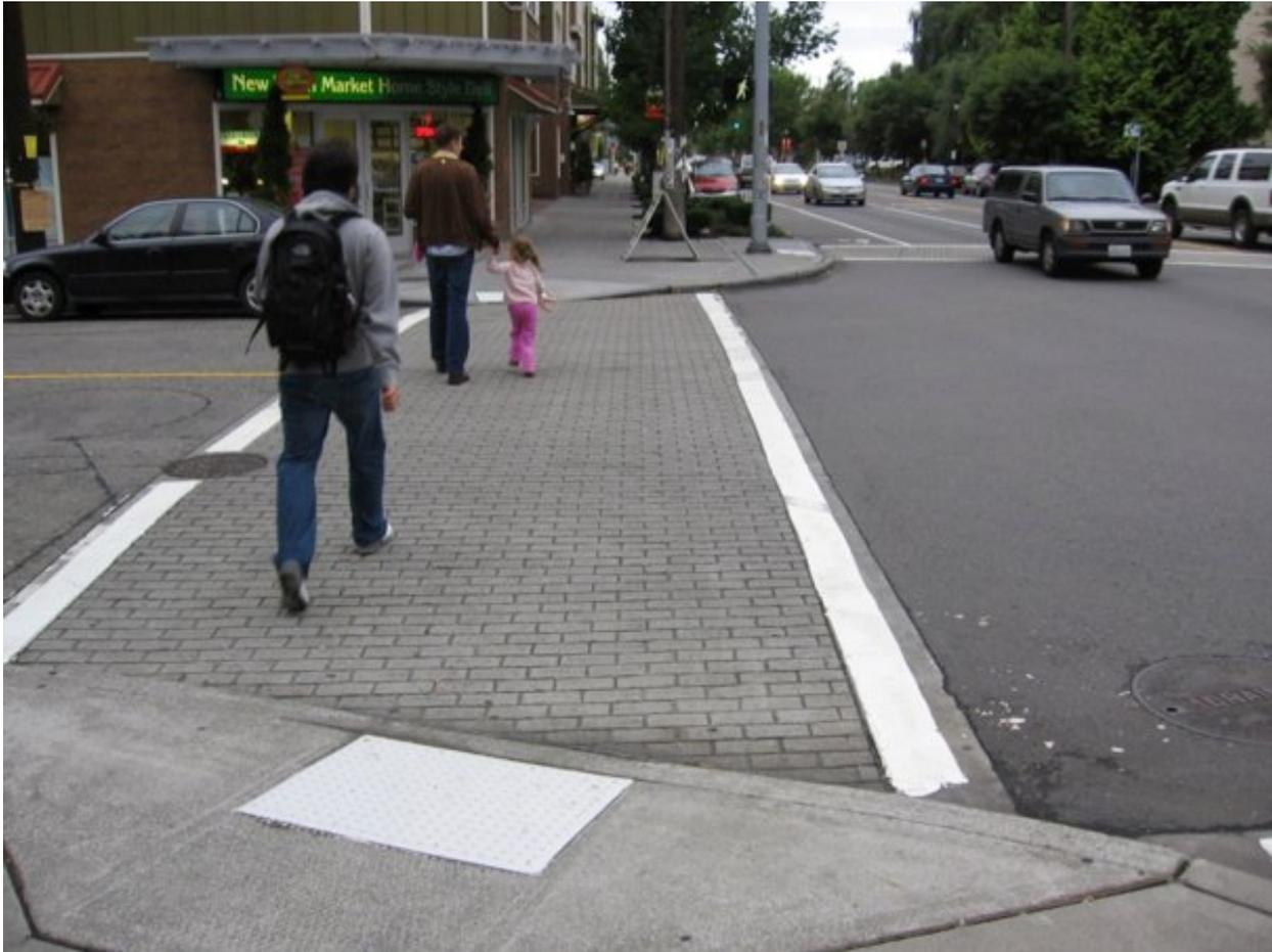
Textured pavement may be used to indicate pedestrian crossings and enhance the pedestrian environment at intersections.
