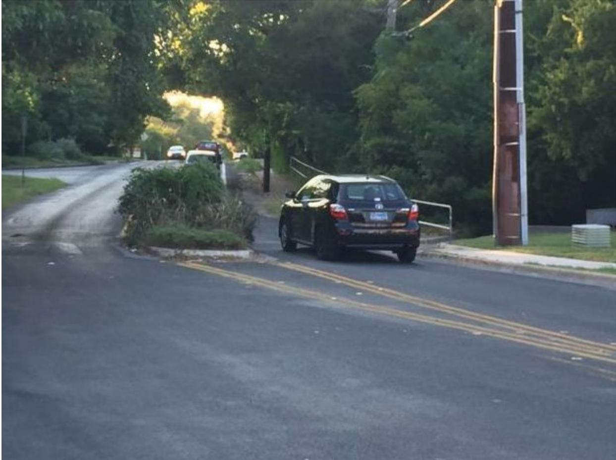
Center-islands create a small amount of deflection in the roadway alignment and reduce the roadway width, reducing vehicular speeds as they navigate through the center-island narrowing.
