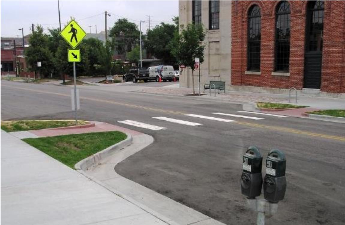
Chokers and Bulb-Outs extend the curb of the roadway, reducing vehicular speeds as they navigate through the reduced roadway width.
