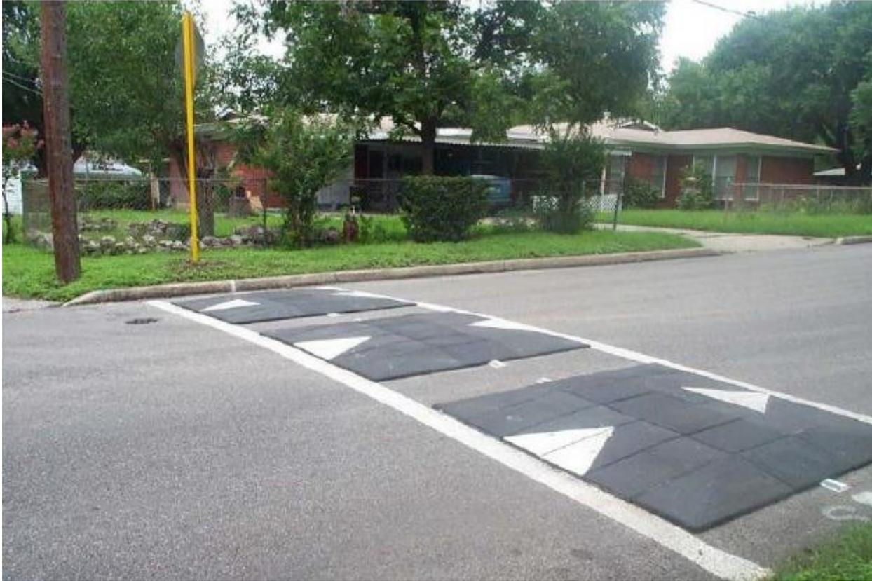
Speed cushions create raised sections on the roadway, reducing passenger car speeds while providing wheel cutouts for larger vehicles.
