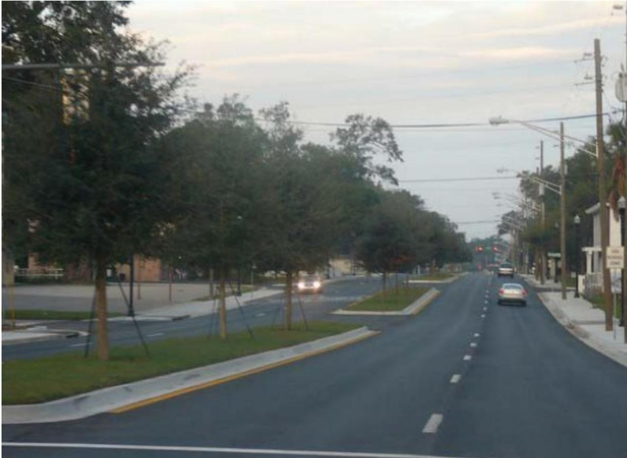
Median barriers are raised islands placed in the center of a roadway between opposing travel directions. These can prevent left-turns from and onto the roadway, reducing conflict points.
