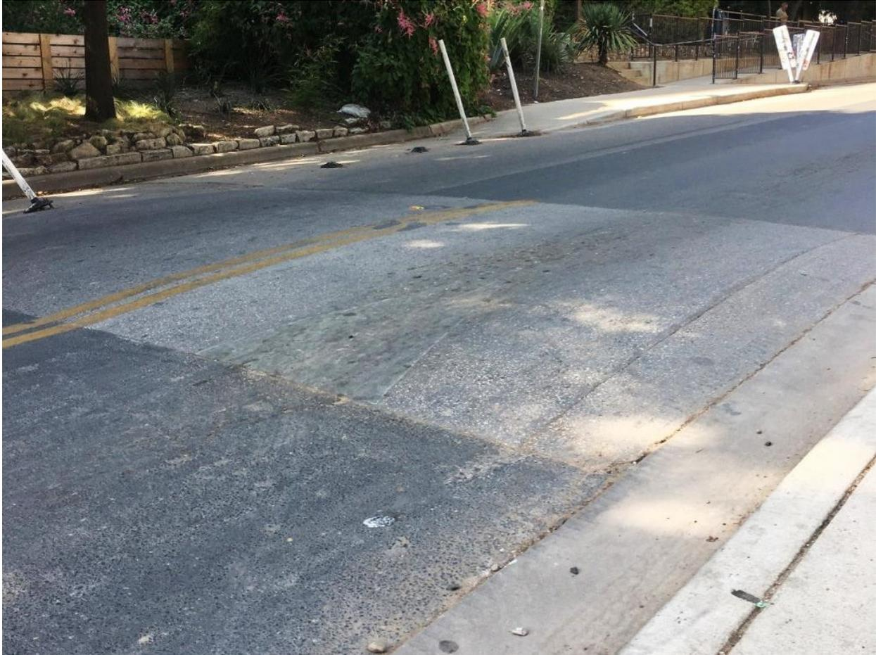
Speed humps create a raised section of pavement across the entire roadway, reducing vehicular speeds.
